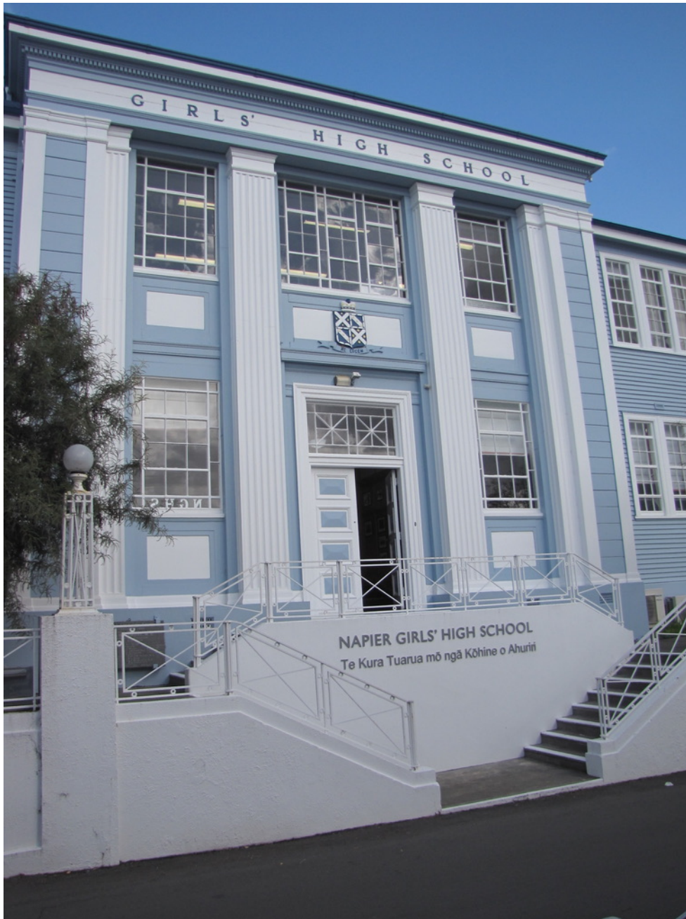
Figure 79 The central bay of the Main Block, notable for its restrained Classical design. The steps rise straight from the street, with no footpath. Source: Chris Cochran May 2019
