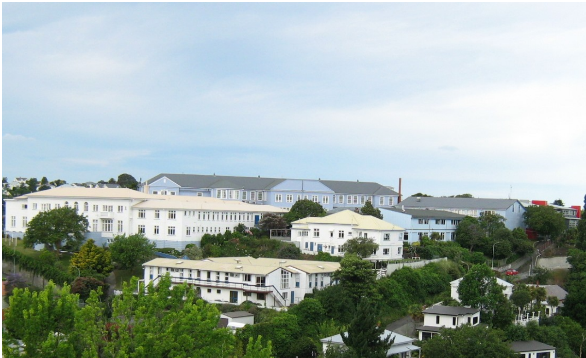
Figure 89 View of Napier Girls' High School showing rear of Main block on skyline. Source: By Kiwichris - Own work, CC BY-SA 4.0, https://commons.wikimedia.org/w/index.php?curid=42866431
