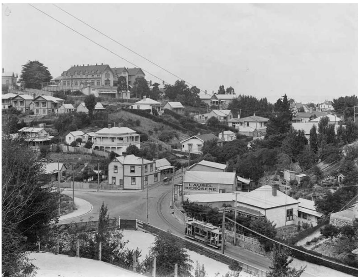
Figure 85 The original school building (on the site of the present hostel) sometime between 1911 and 1931. Source: MTG Hawke's Bay Object nos. m59/23, 2352, 91903
