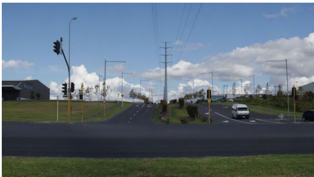
Figure 6: Highbrook Development in South Auckland
