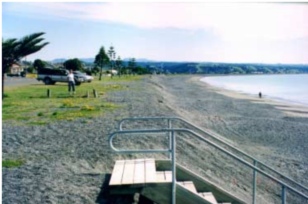
• Plate 5: Photograph taken 28 September 2001 by Dr Gibb looking North along the artificial embankment constructed and maintained along The Esplanade since January 1987.
