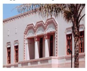
Balconies and small first floor galleries are another feature of heritage buildings in Napier, varying in detail across Art Deco, Spanish Mission and Stripped Classical styles. Some balconies are lightweight, supported on wrought iron or concrete brackets and with delicate wrought iron railings. Others are more substantial features perhaps with balustrades resembling stone or concrete. Iron railings
