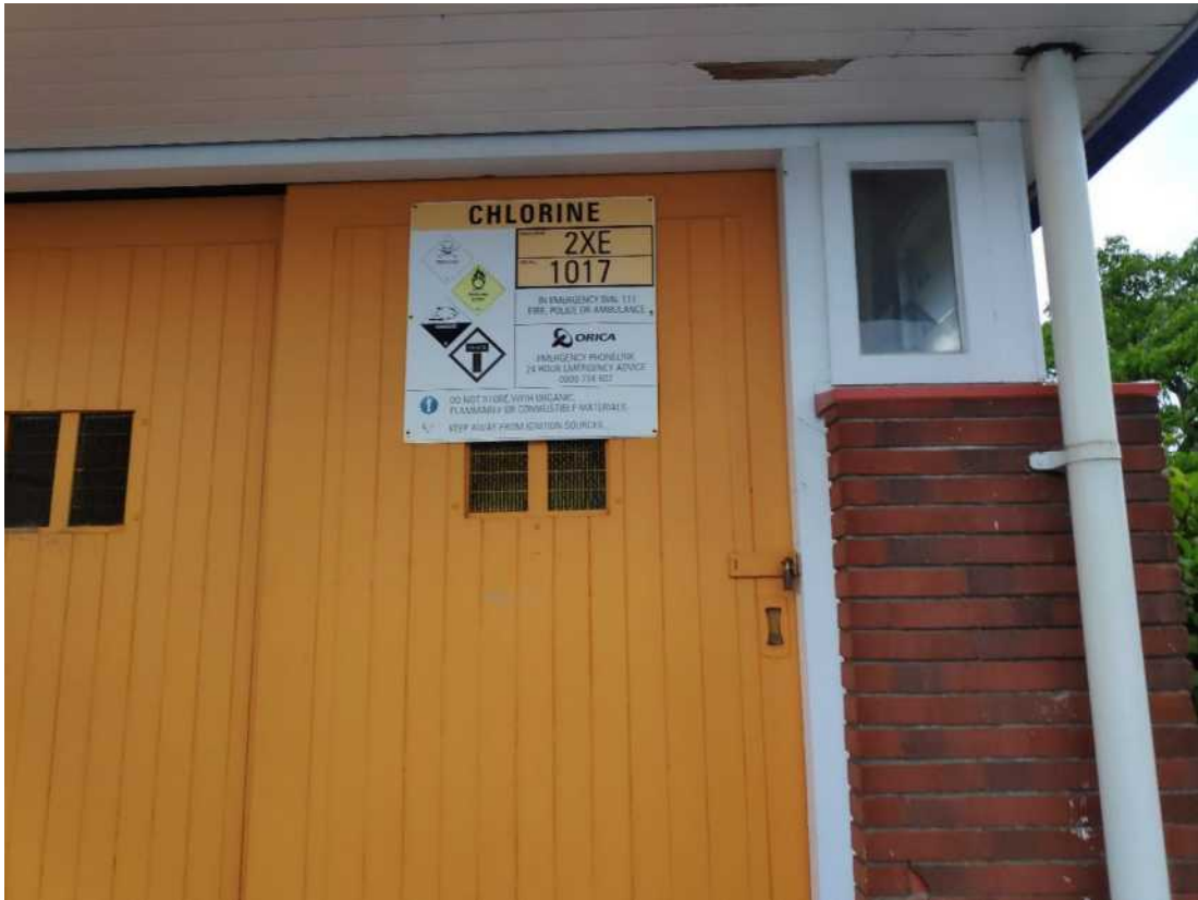
Photograph 7: Hazardous storage shed.
