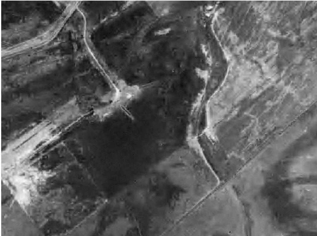
Historical Aerial Image 1: 1936, sourced from NCC.
