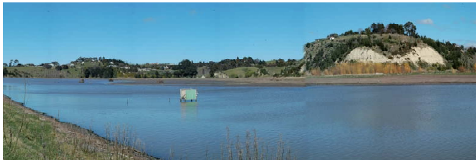
Figure 39: Middle Estuary (Main Outfall Channel) from SH2 Expressway
