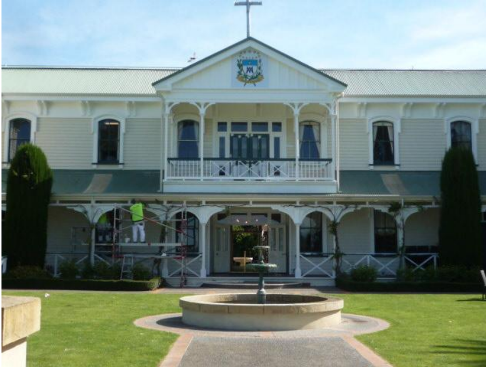
Plate 4. La Grande Maison, central section. Image: D.Harlow Oct 2016 Maintenance is ongoing.
