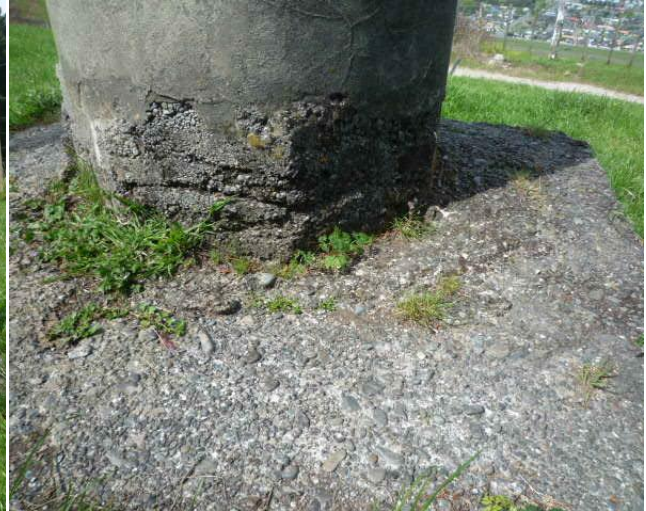
Plate 14. Stream pebbles used in the construction of the base and pedestal.
