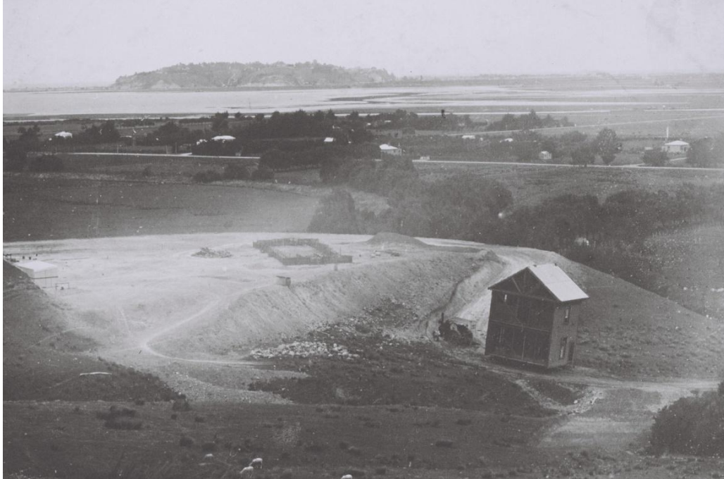
Plate 1. Greenmeadows 1911. A platform formed for the Mission building, 'La Grande Maison', which had been cut into eleven sections for transportation to the site. Church Road in the middle distance. Scinde Island in far distance. Marist Archives, Courtesy: Peter Holley
