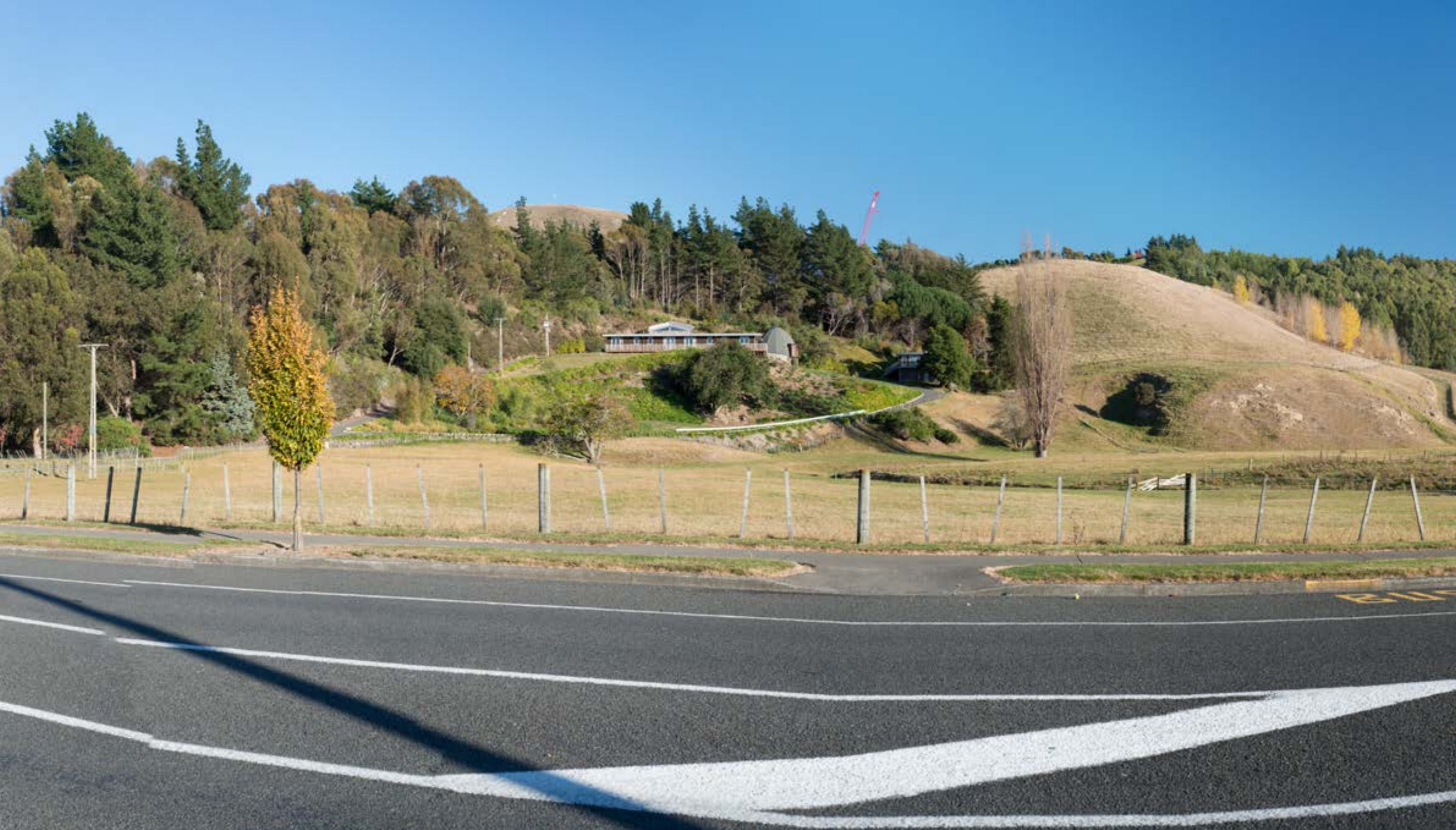
Figure 19. Before and after photomontage from Church Road viewpoint A (before) View from Church Road looking towards the Mission Landscape
