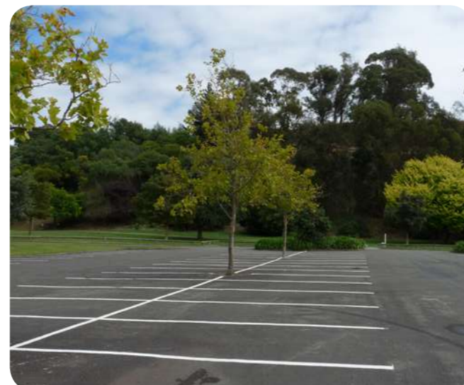
During mid-week there are very few cars and car parks are large areas of asphalt.
