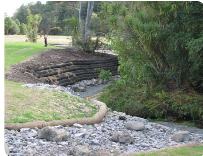
Lucas Creek, Auckland: Just after earthworks and formation
