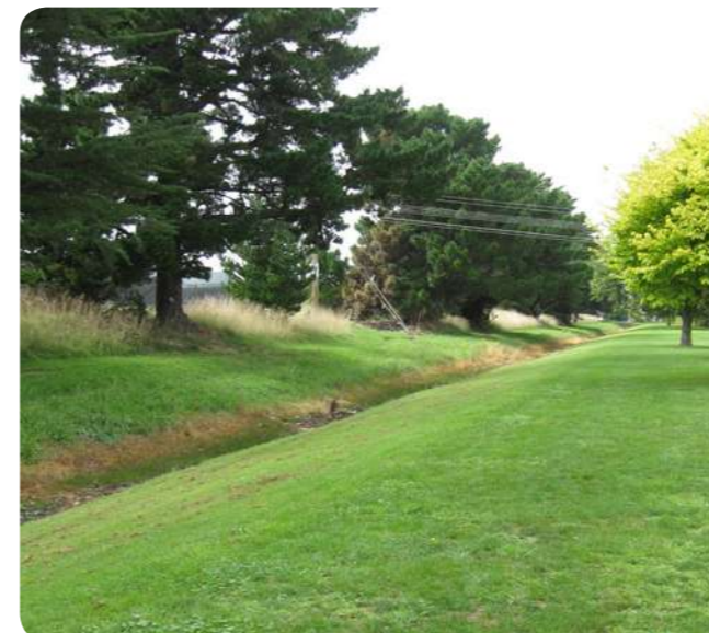
As Park Island is low lying and was formally part of Ahuriri Estuary there are several drains through the park with banks that are mown right to the edge.
