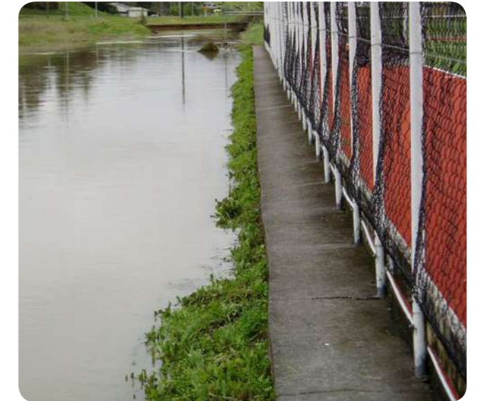
Taipo Stream flooded April 2011, water level close to over-spilling on to Hockey Turf.
