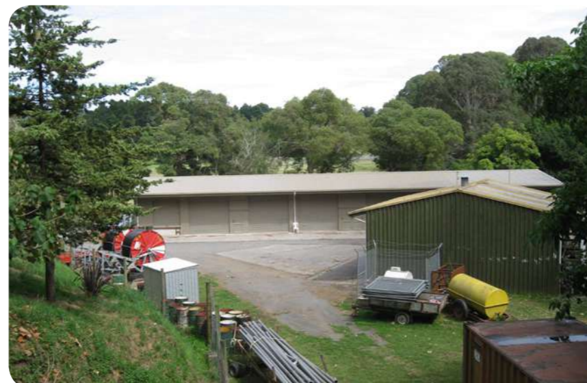
Napier City Council Depot and yard.
