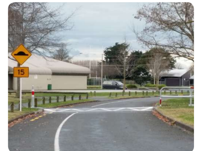
Raised table crossing
