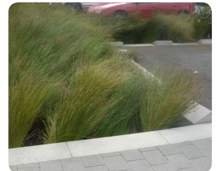
Rain gardens in car park areas.
