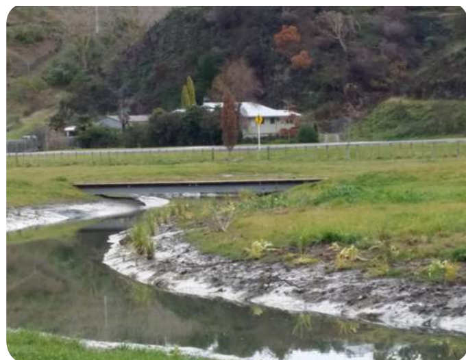
Taipo stream just after earthworks and formation
