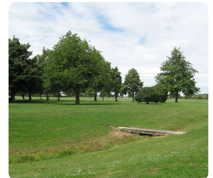
Wooden platforms over drains allows access between areas.
